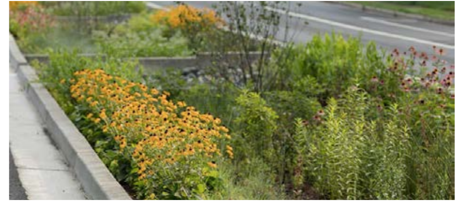
THE AVENUE PLANTED RAINGARDENS
