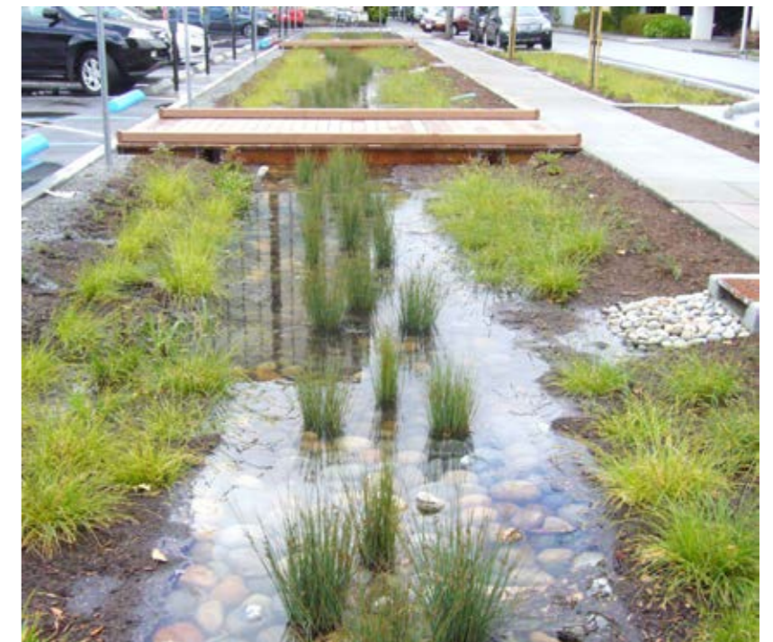
RAINWATER ACCUMULATION IN RAINGARDEN
