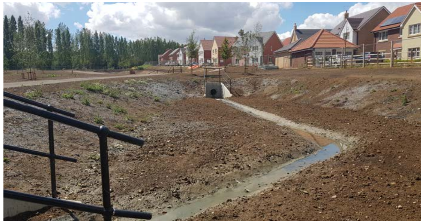
ATTENUATION BASIN (DAVENTRY) – AT CONSTRUCTION
